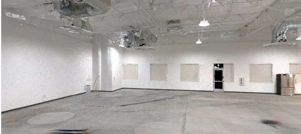
Figure 2: This represents the interior scan quality of the FARO S150.
