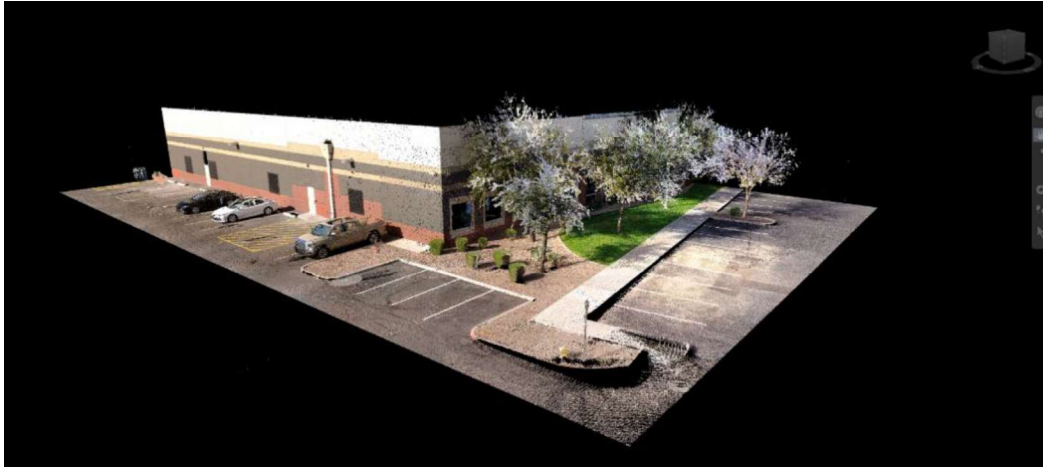
Figure 5: This small section of the exterior scans highlights accurate colorization for the FARO scanner and crisp surfaces. Please see reference image on right to compare with actual conditions.
