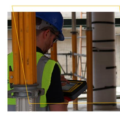
"Using (a) robotic total station, we set approximately 500 individual field points in one day with one person. Comparable conventional methods using a tape measure would have taken several days. When it comes to concrete deck insert layouts, we have increased our productivity by a factor of 10.
